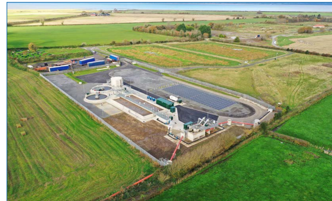
Ballykelly wastewater treatment works, County Derry/Londonderry.
