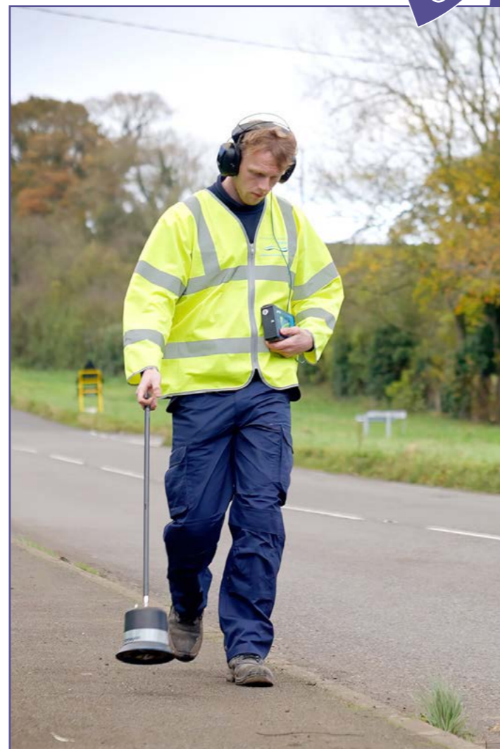
Detecting leaks using a ground microphone.
