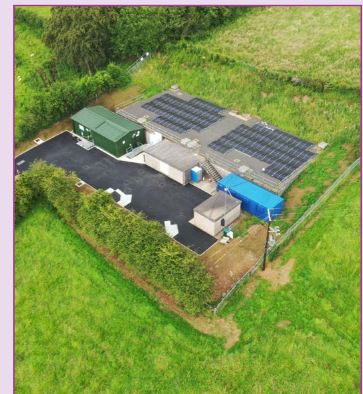
Moneymore Borehole in County Derry/Londonderry.
