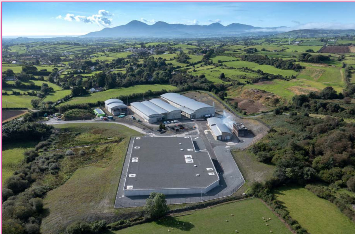
Completion of the £13m investment at Drumaroad water treatment works in County Down to benefit a quarter of Northern Ireland's population.
