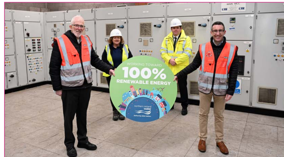
Piloting the production of green hydrogen - NI Water staff showing Alliance Party of Northern Ireland MLA's Andrew Muir MLA and Stewart Dickson MLA the 10kW Electrolyser at Kinnegar Wastewater Treatment Works in Belfast.
