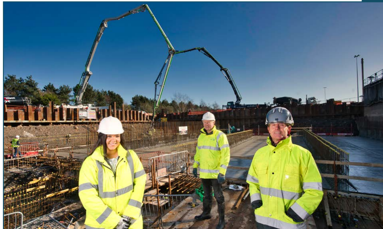
Construction of new treatment tanks at Belfast wastewater treatment works.
