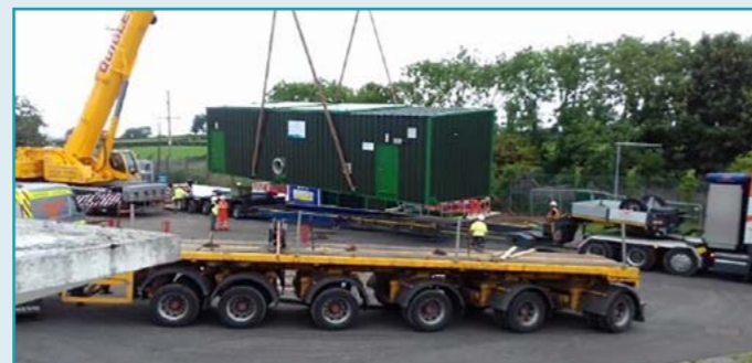
Installation of the modular pumping station.
